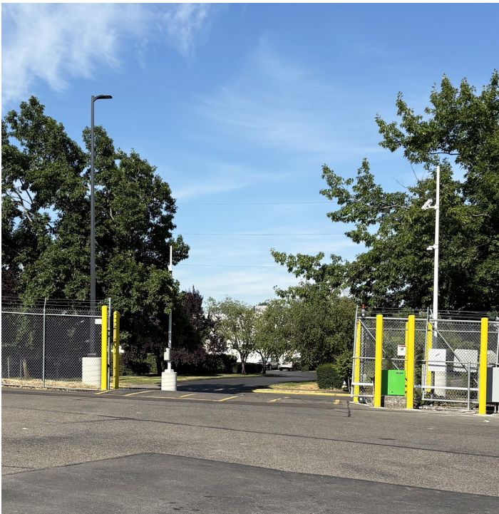
Figure 2. Unsecured Truck Entrance
