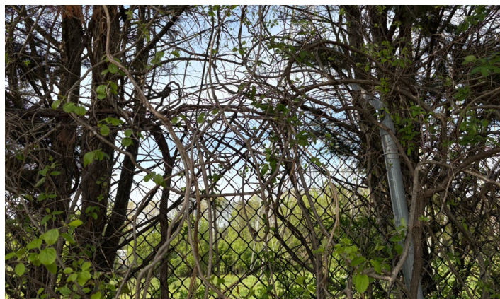
Figure 5. Damaged Fence and Overgrown Trees
