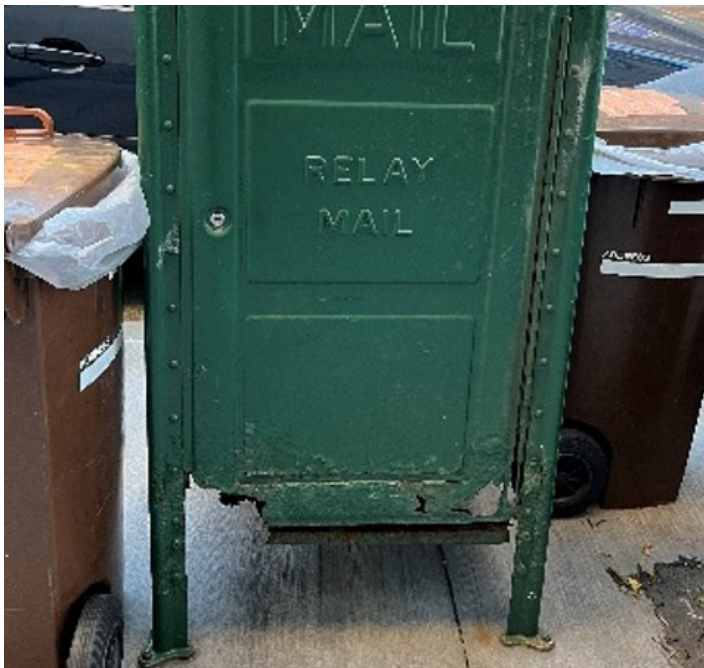
Figure 5. Green Relay Box with HSEL and Rusted-Through Hole at the Bottom
