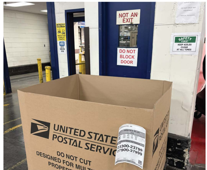
Figure 10. Examples of Blocked Access to Observation Door and Fire Alarm
