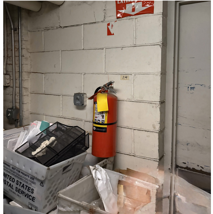
Figure 3. Basement Boiler Room Fire Extinguisher blocked by MTE
