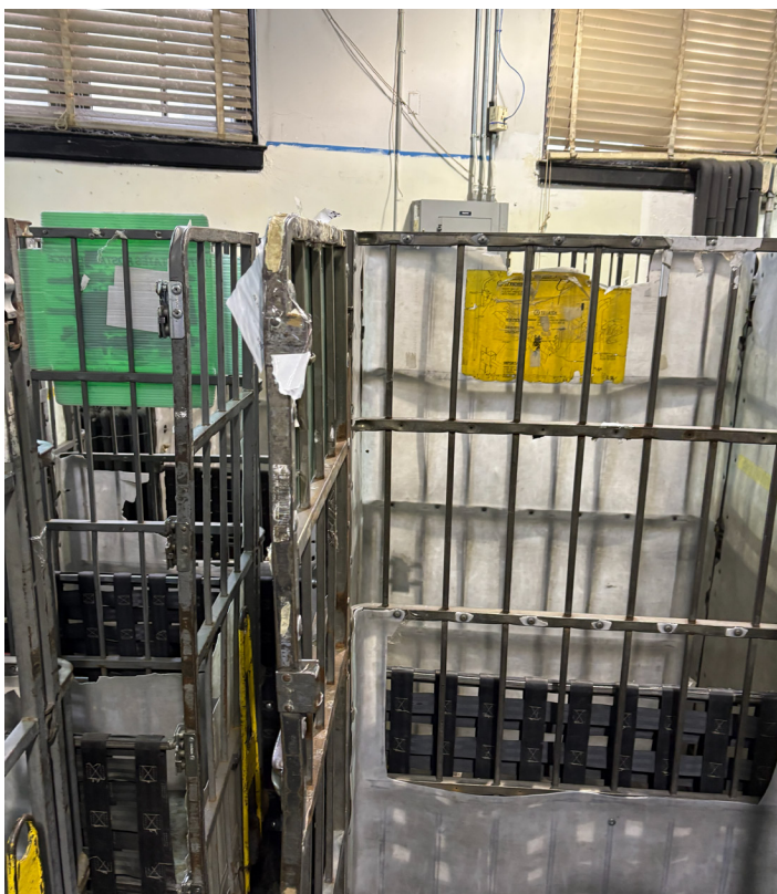
Figure 4. Blocked Electrical Panels in Workroom Area
