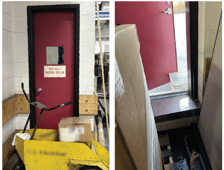
Figure 3. Examples of Blocked and Propped Open Doors
