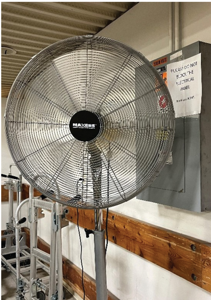
Figure 3. Blocked Electrical Panel
