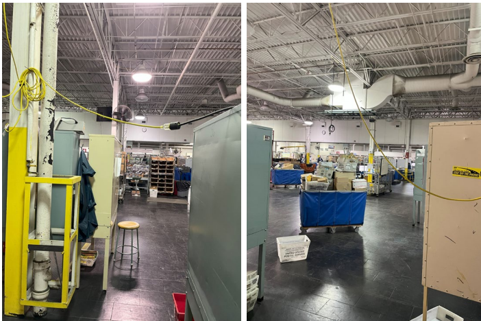
Low Hanging Wires on the Workroom Floor
