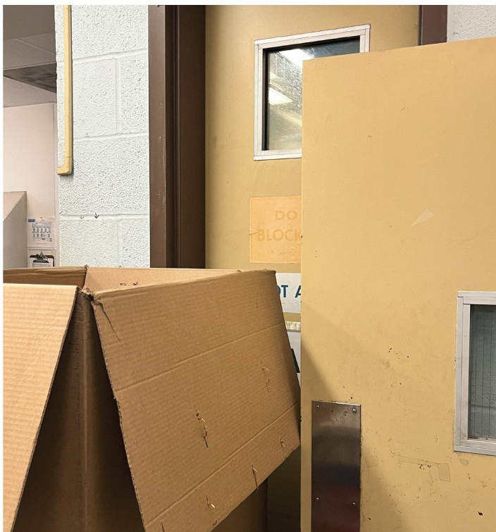
Blocked Inspection Service Door
