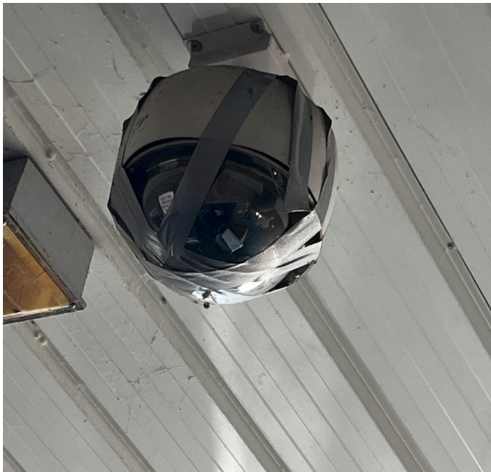
Figure 3. Camera Cover Held On With Tape
