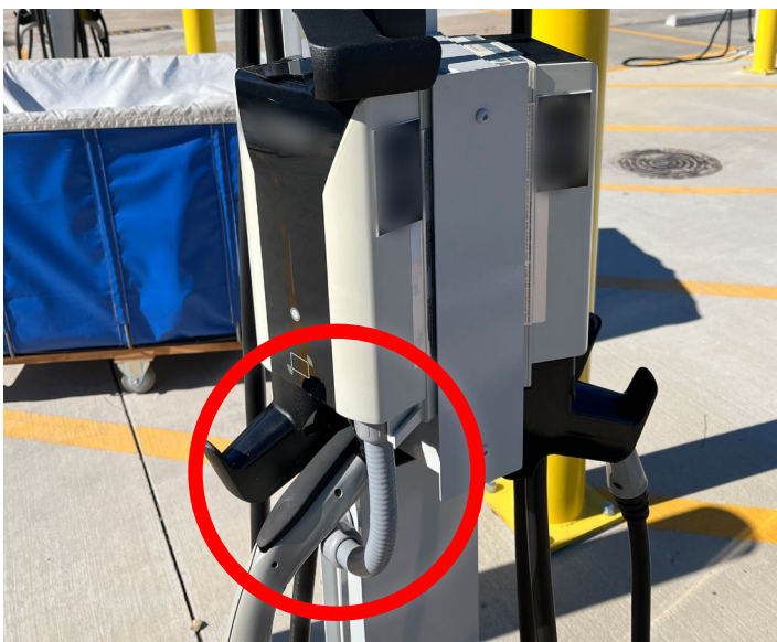
Figure 6. Missing Hook (red) vs. Undamaged Equipment (blue)
