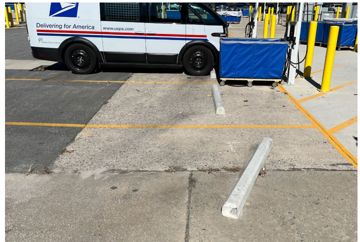
Figure 4. Misaligned Wheel-Stop Placement
