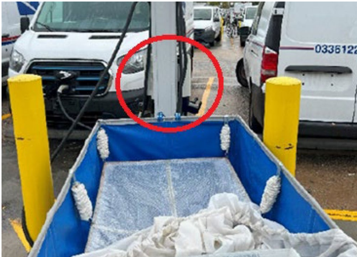
Figure 5. Inadequate Bollard Protection for Charging Station (in red)
