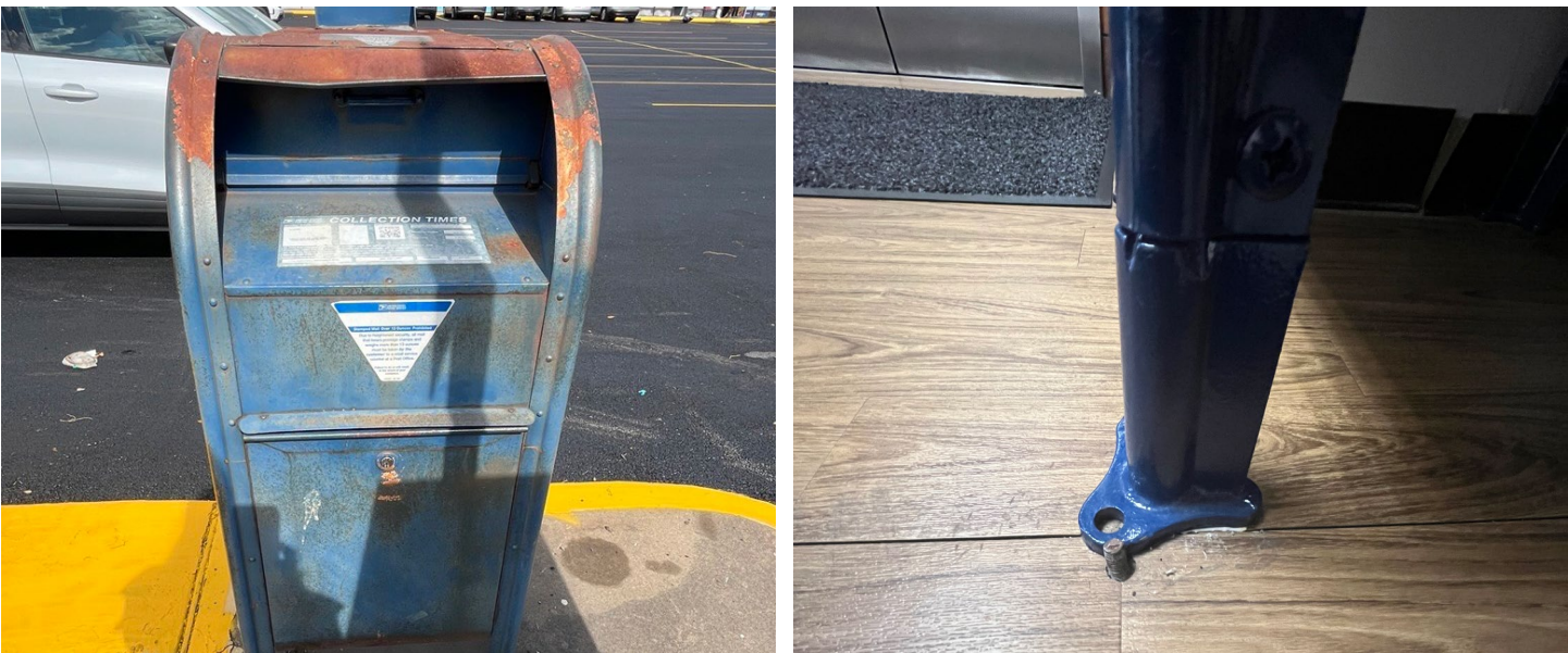
Figure 8. Houston, TX, Blue Collection Box With Corrosion and Missing Leg Bolt
