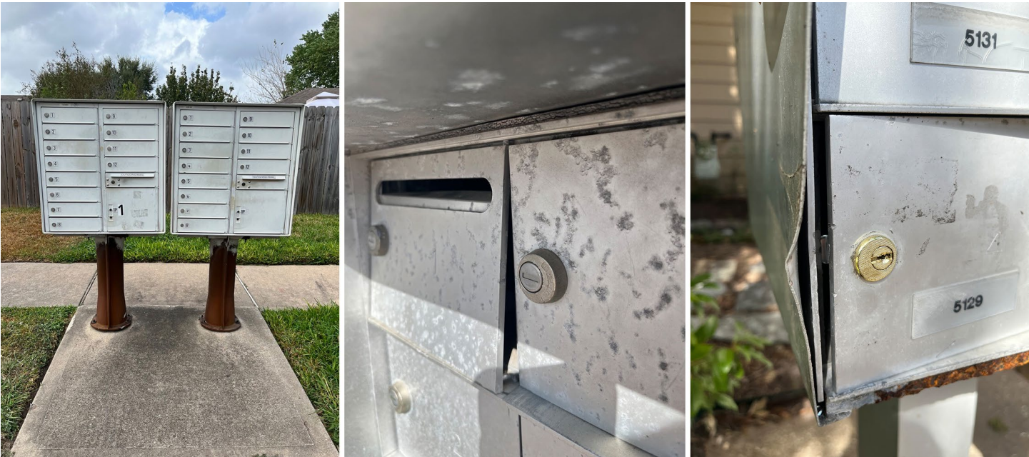
Figure 9. Houston, TX, Cluster Box Unit With Corrosion and Door Gap
