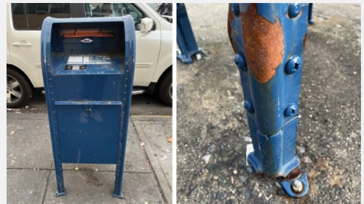
Blue collection box with missing bolts and corrosion seen in Queens, NY, during mail theft mitigation audit. Source: OIG photograph.
