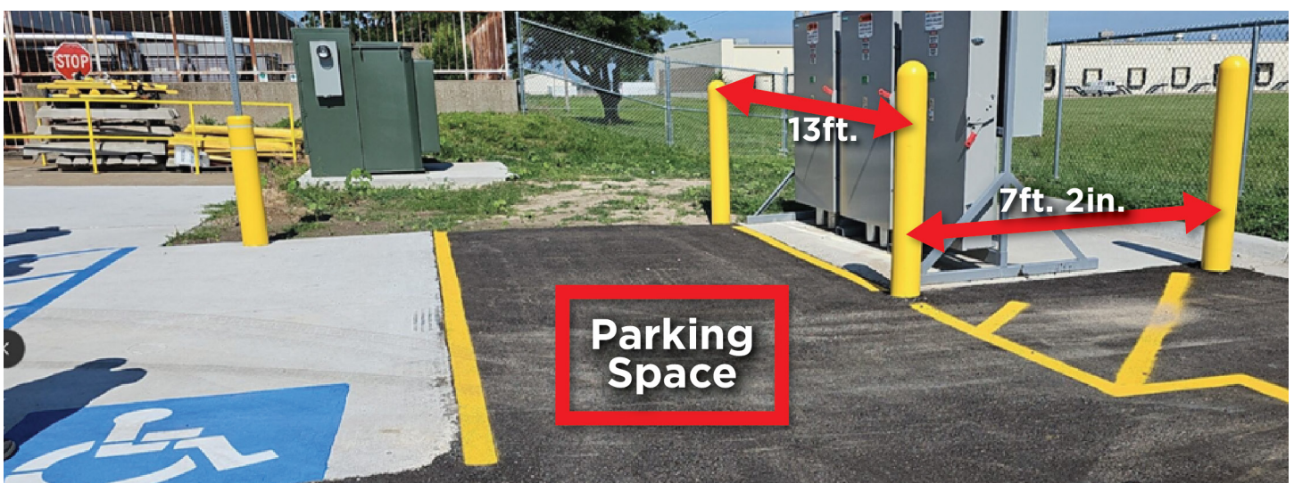
Figure 6. Insufficient Number of Bollards Near Electrical Panels
