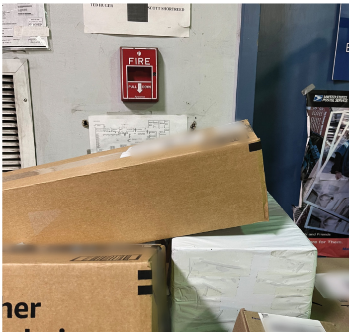
Figure 5. Blocked Manual Fire Alarm Pull at Mount Pleasant Post Office
