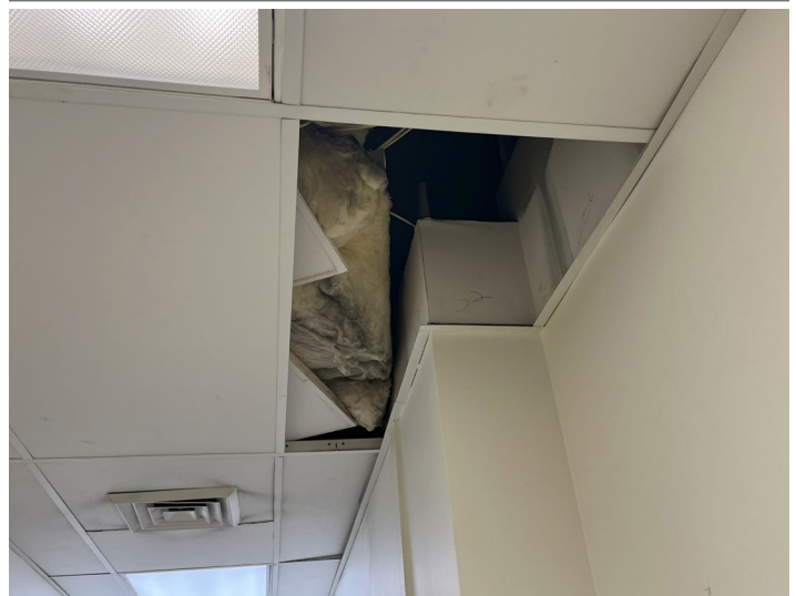
Figure 6. Missing Ceiling Tile
