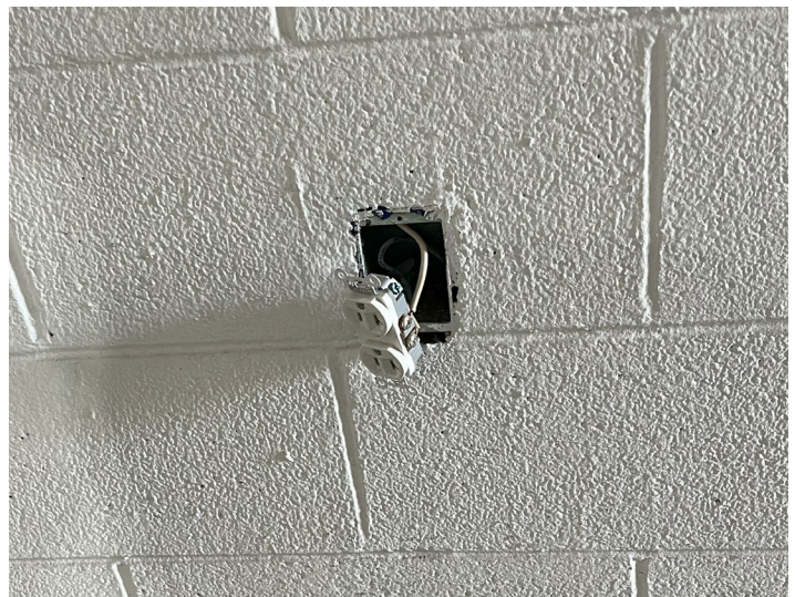
Figure 5. Broken Electrical Outlet
