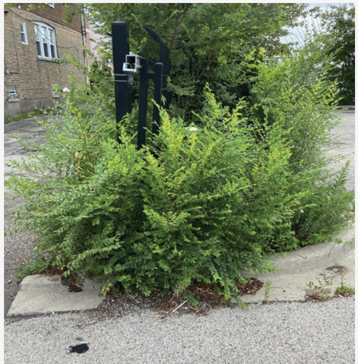
Figure 9. [REDACTED] Gate Blocked by Overgrown Brush
