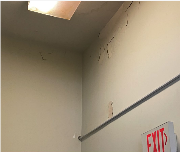
Figure 3. Examples of Peeling Paint
