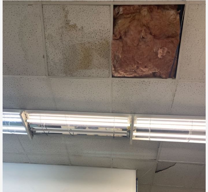
Figure 4. Example of Stained and Missing Ceiling Tiles
