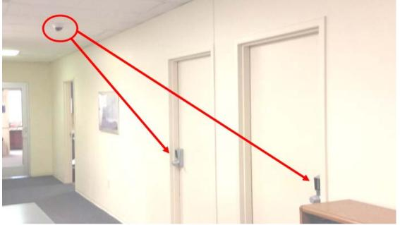
Figure 2. Surveillance Camera Observing Combination Lock Doors
