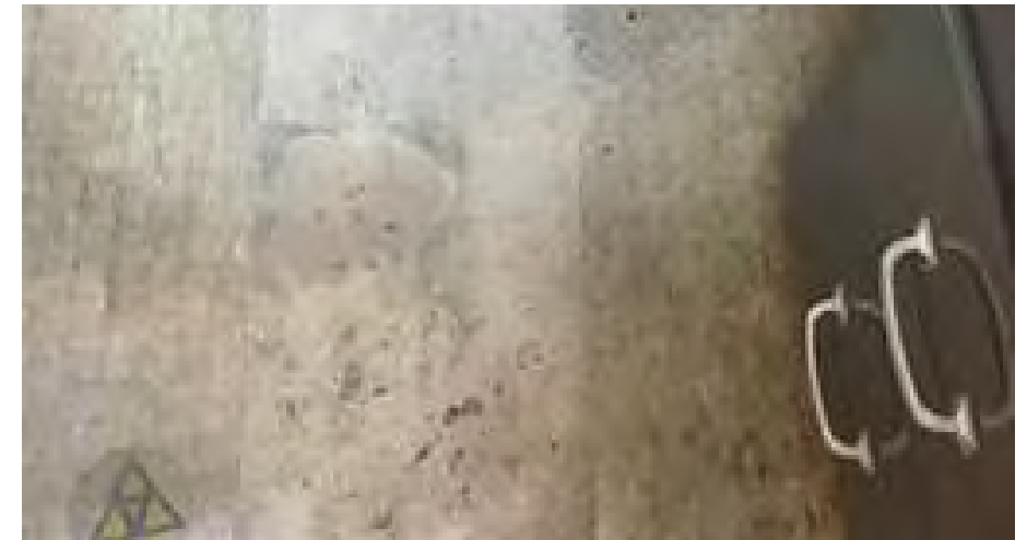
Figure 9: Damaged Asbestos Floors
