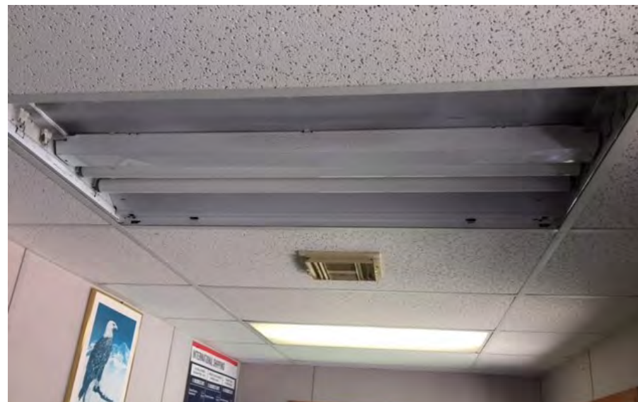
Figure 4. Bulbs Need Replacement and Cover is Missing
