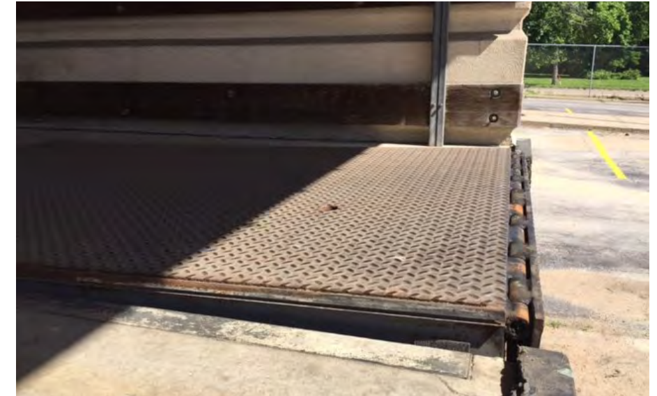
Figure 5. Tripping Hazard – Uneven Loading Dock Plate
