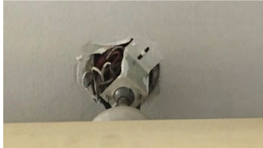
Figure 6. Exposed Wiring
