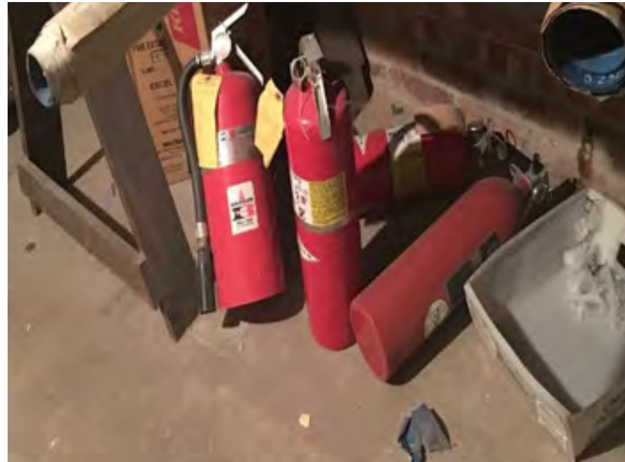
Figure 2. Inoperable Fire Extinguishers
