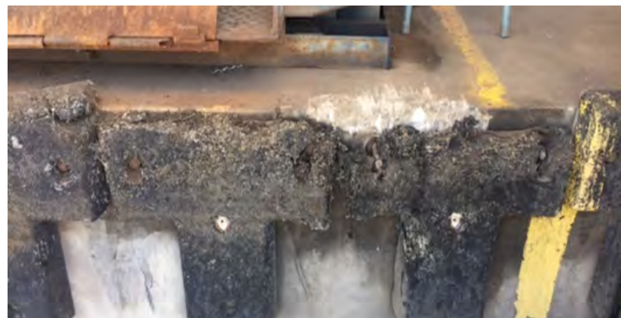
Figure 10. Damaged Loading Dock Bumper
