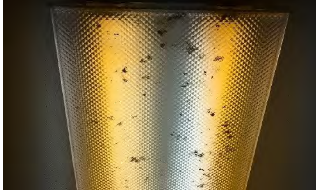
Figure 12. Dead Bugs in Ceiling Light Fixture
