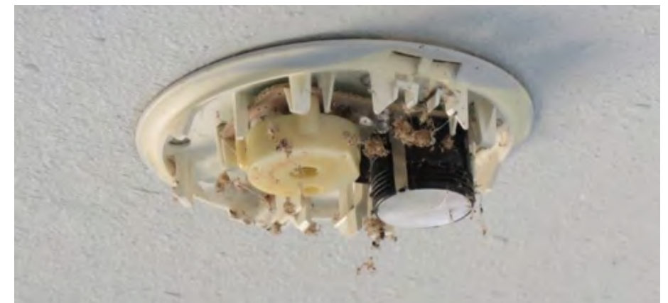
Figure 8. Inoperable Smoke Detector
