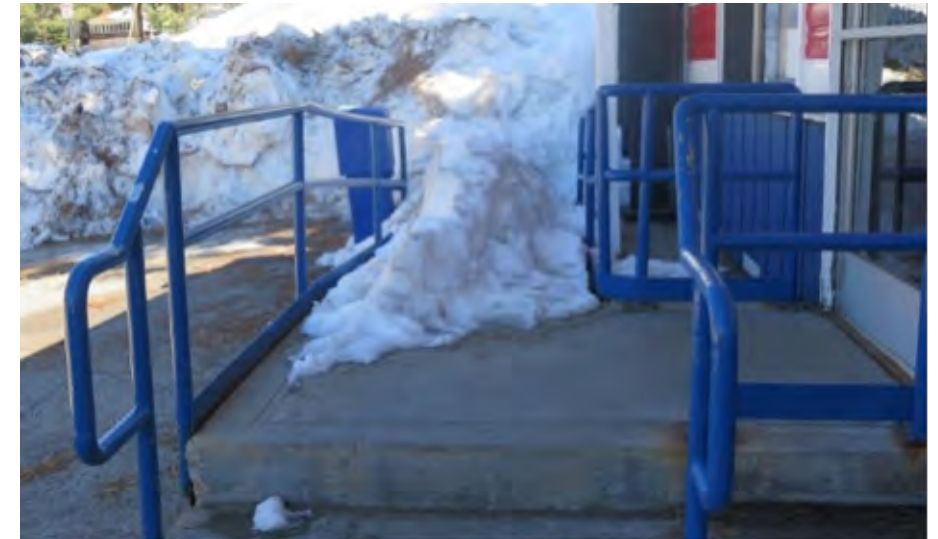
Figure 13. Obstruction of Handicap Accessible Ramp
