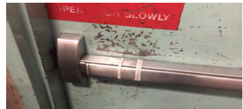
Figure 1. Altered Locking Mechanism on Exit Door
