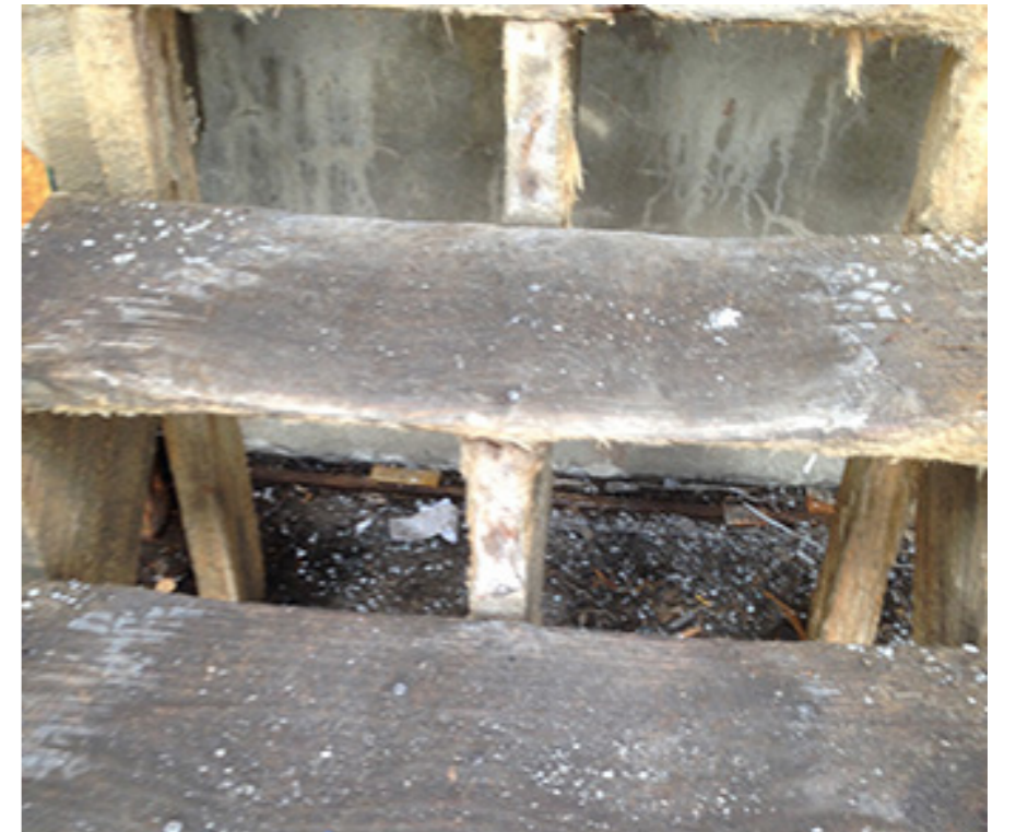
Figure 10: Warped Stairs
