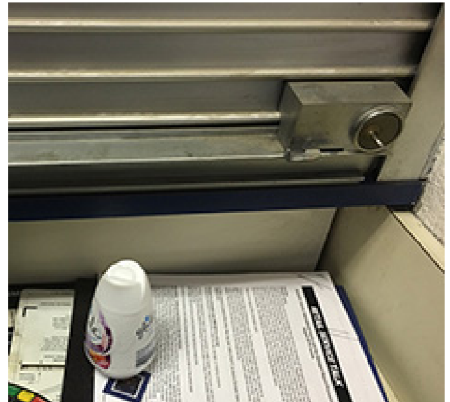
Figure 2: C-Clamp Securing Retail Counter
