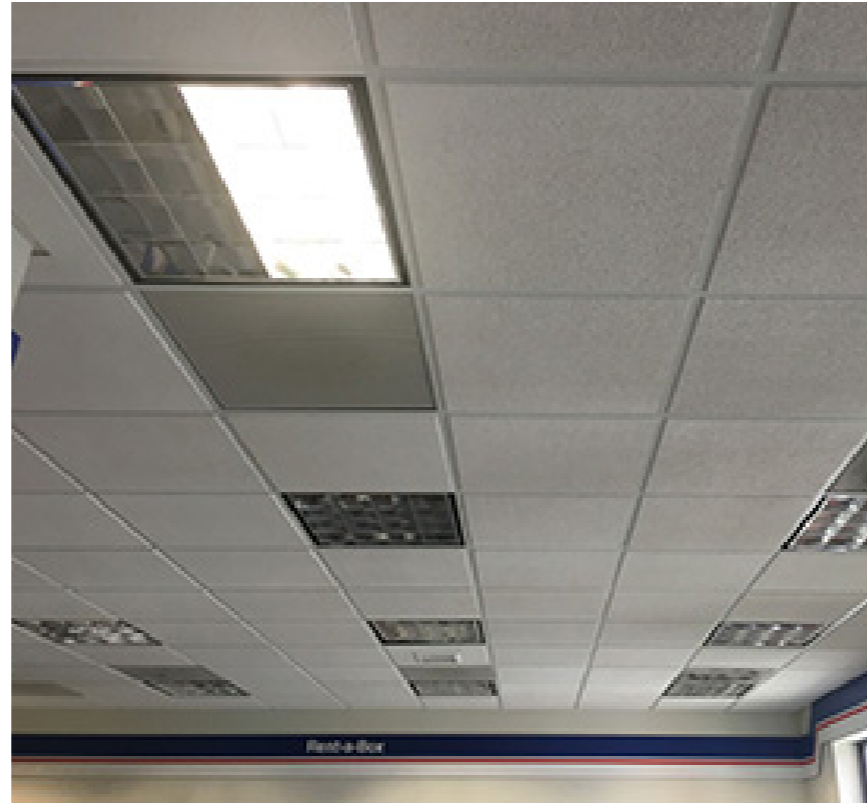
Figure 5: Missing Bulbs
