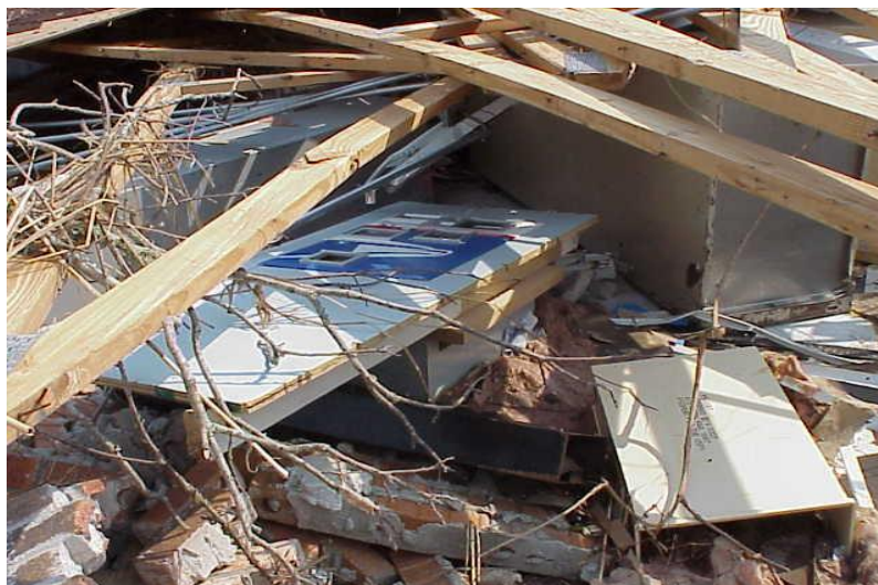
Damaged Postal Service Facility—Photograph 4 11
