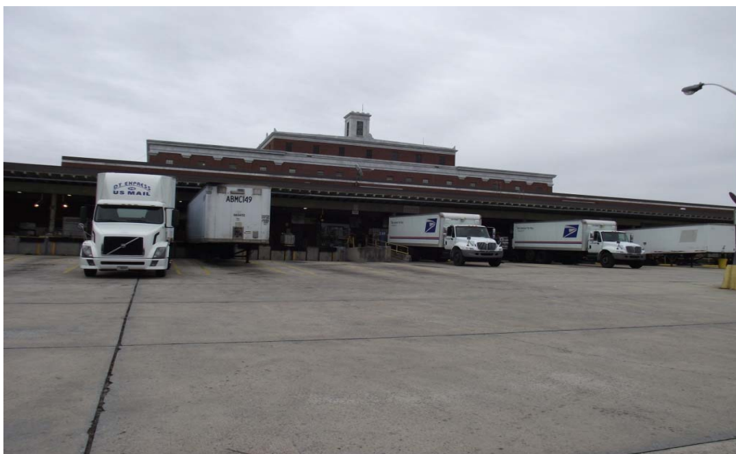
Source: OIG Illustration 4: Macon P&DC has 27 dock doors. Additional dock doors allow for more efficient dock operations and reduce congestion. Photograph taken December 15, 2010.
