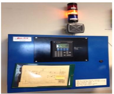
Figure 1 – Methane Detection System Main Control Panel
