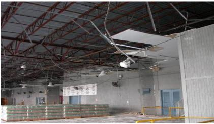
Figure 2. Collapsed Ceiling at the Gulfport P&DF
