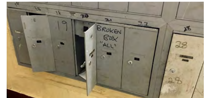
Figure 5. Broken Mailboxes at a Building
