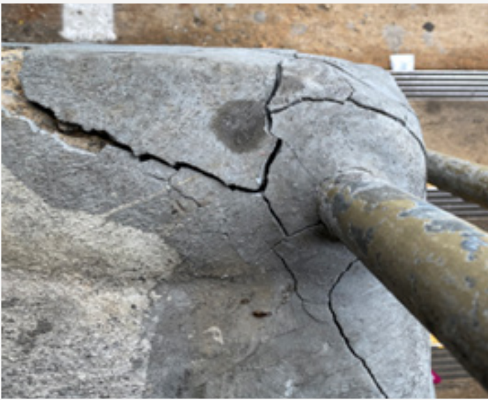
Figure 7. Cracked Concrete
