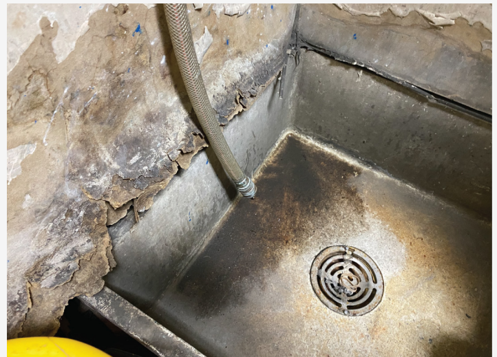
Figure 5. Damaged Walls at the Custodian Sink
