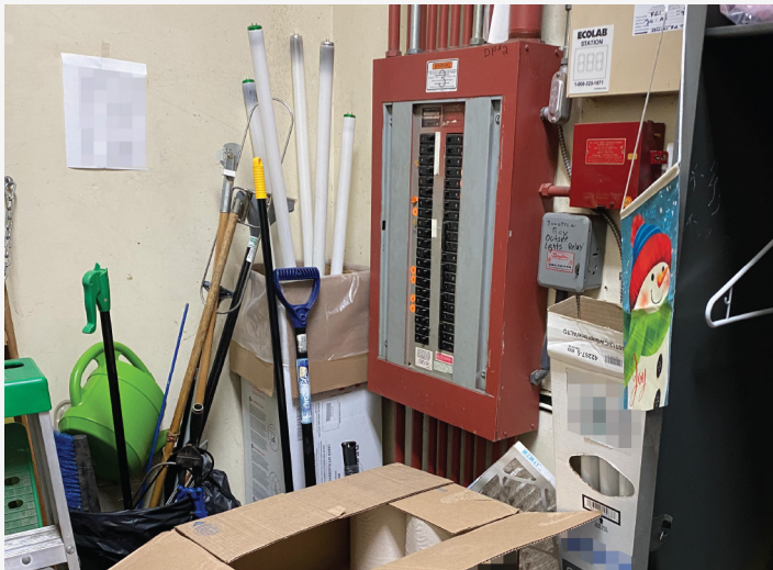
Figure 4. Blocked Electrical Panel
