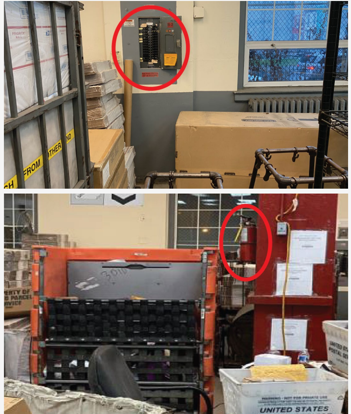
Figure 4. Blocked Electrical Panel and Fire Extinguisher
