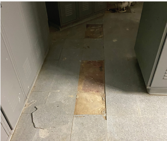
Figure 3. Missing Floor Tiles in Men's Locker Room
