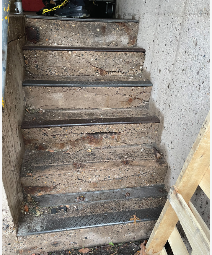
Figure 4. Damaged Dock Staircase with Multiple Tripping Hazards
