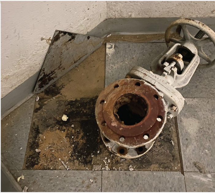
Figure 6. Evidence of Potential Mold in Men's Locker Room
