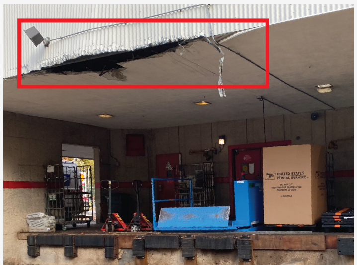
Figure 5. Large Opening in Roof Above Dock
