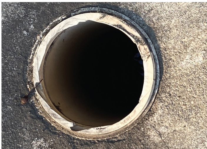
Figure 5. Uncovered Drainage Hole in Postal Vehicle Lot at Stockbridge MPO
