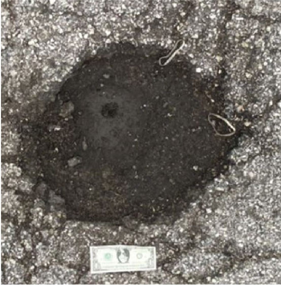
Figure 4. Pothole in Employee Parking Lot
