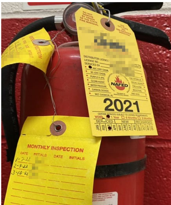
Figure 1. Example of Fire Extinguisher Missing Inspections
