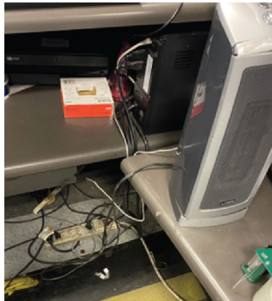
Figure 2. Space Heater Plugged into Surge Protector
