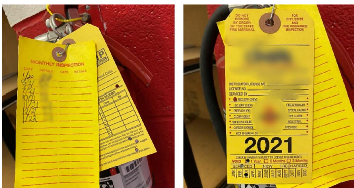
Figure 9. Examples of Expired Fire Extinguisher Inspections
