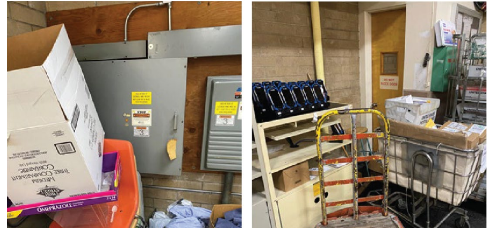
Figure 1. Blocked Electrical Panel and Inspection Service Door
