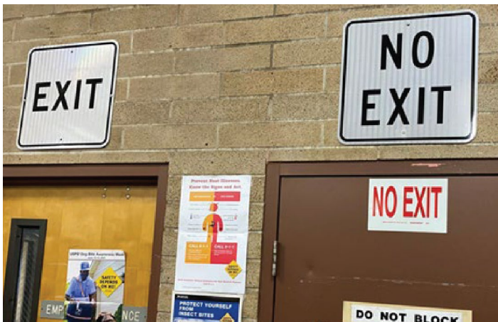
Figure 4. No Illuminated Exit Signs
