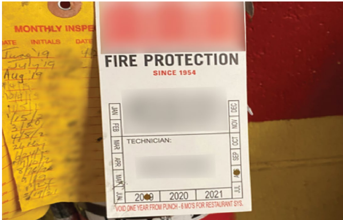
Figure 3. Portable Fire Extinguisher Missing Annual Inspections
