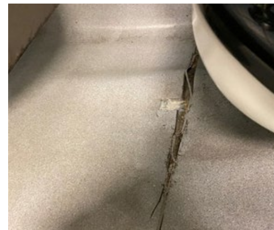
Figure 6. Cracked Flooring in Men’s Restroom
