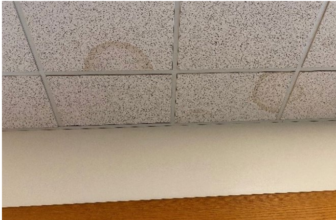
Figure 11. Stained Ceiling Tiles in the Lobby
