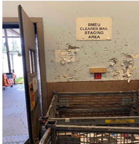
Inside Dock Area
