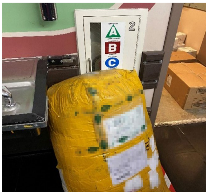
Figure 2. Blocked Fire Extinguisher
