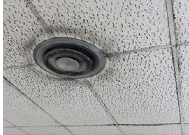
Figure 13. Dust Around Air Vent
