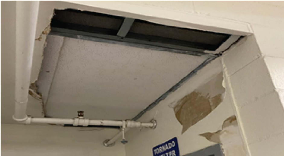
Figure 8. Hole in Ceiling
