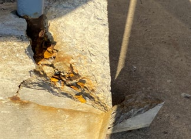
Figure 5. Damaged Concrete
