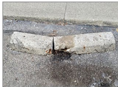
Damaged/Misaligned Wheel Stops
