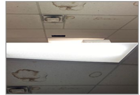
Stained Ceiling Tile
