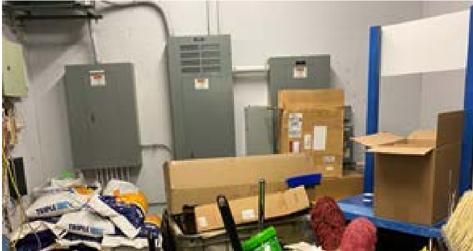
Figure 1. Blocked Electrical Panels
