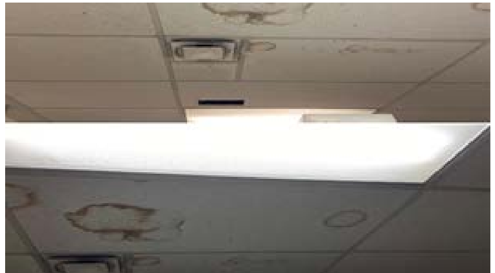
Figure 4. Stained Ceiling Tiles
