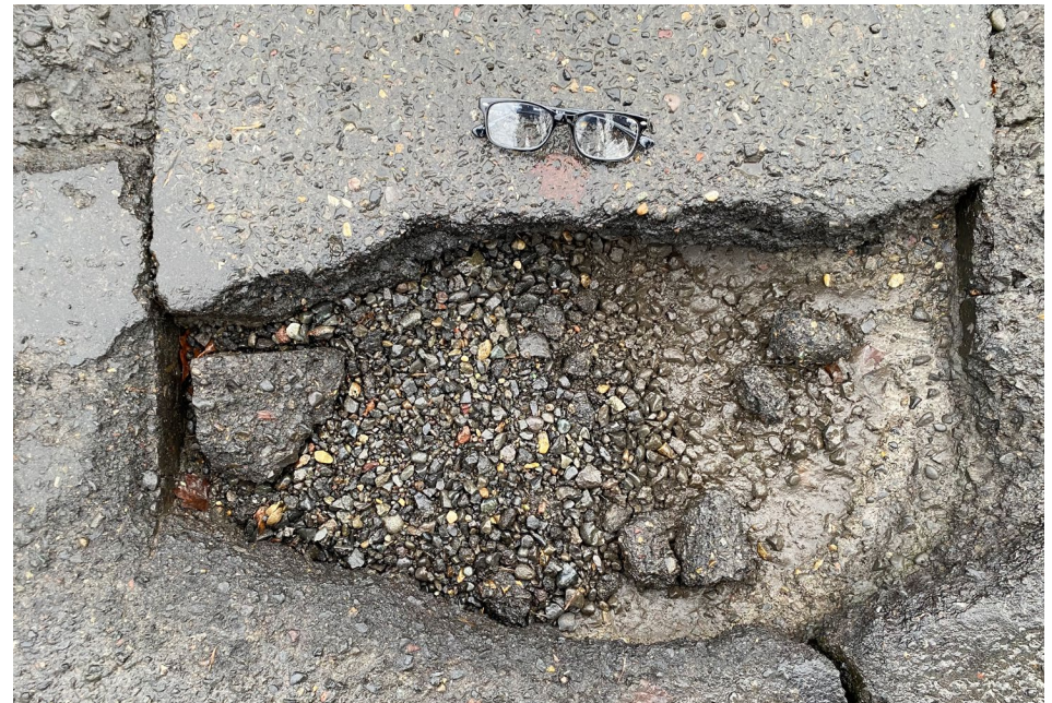
Figure 2. Damaged Asphalt
