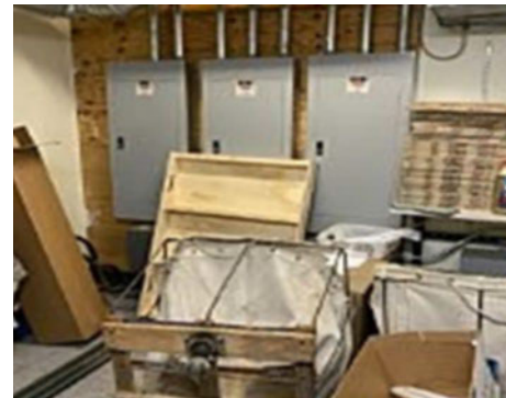
Source: OIG photograph taken October 27, 2021 – blocked electrical panels – New Palestine Post Office.
