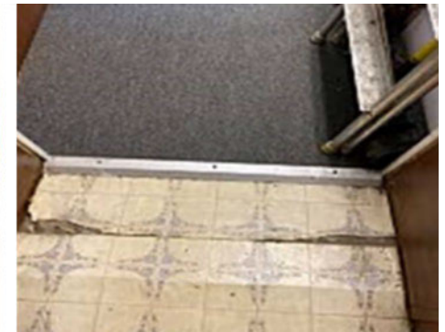
Source: OIG photograph taken October 27, 2021 – damaged vinyl flooring – Maxwell Post Office.
