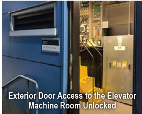
Source: OIG photograph taken during week of February 14, 2022, at Westchester P&DC.
