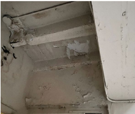
Figure 10. Dirty and Damaged Walls with Potential Mold
