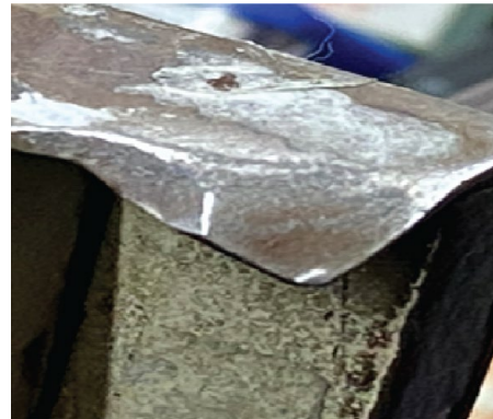
Figure 11. Sharp Edges at Retail Counter
