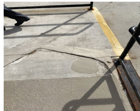
Figure 1. Damaged Ramp
