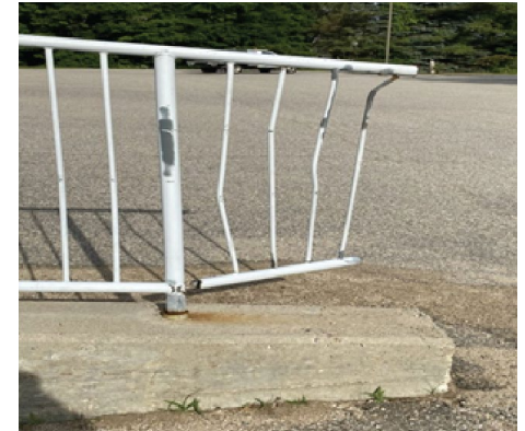
Figure 12. Damaged Handrail
