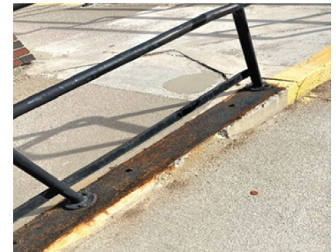
Figure 2. Rusted Handrail
