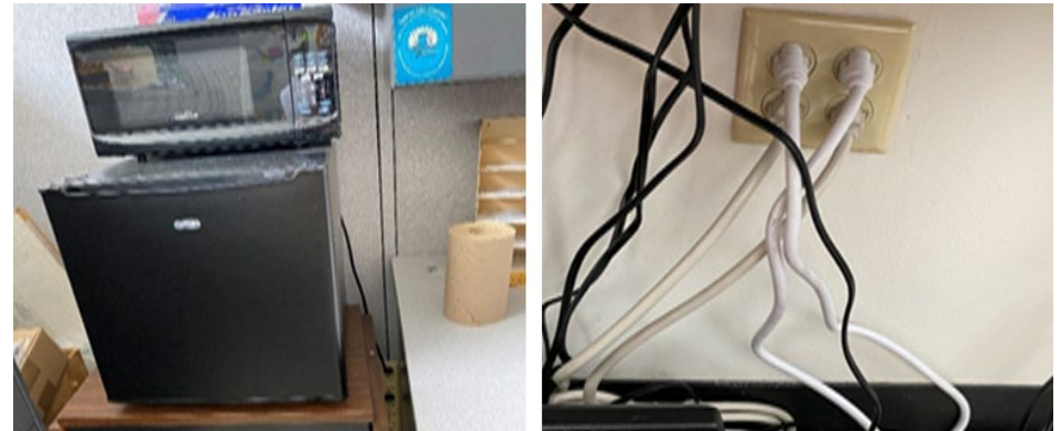
Figure 7. Excessive and Unsafe Power Strip Usage
