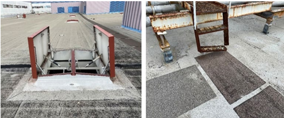
Figure 9. Open Fire Vents and Unsecured Crossover Bridge
