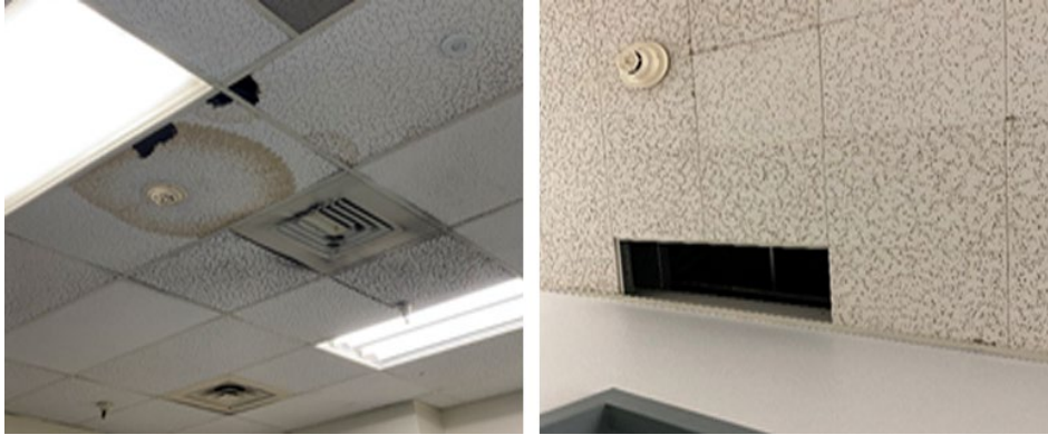
Figure 1. Stained, Broken, and Missing Ceiling Tiles
