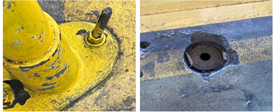
Figure 10. Protruding Bolts and Broken Concrete
