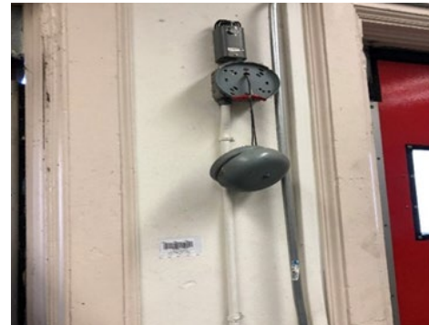
Figure 14. Unsecured Bell Cover
