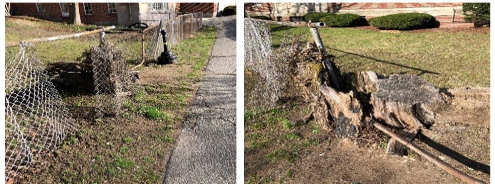
Figure 8. Damaged Chain Link Fence Adjacent to Neighborhood Walking Path
