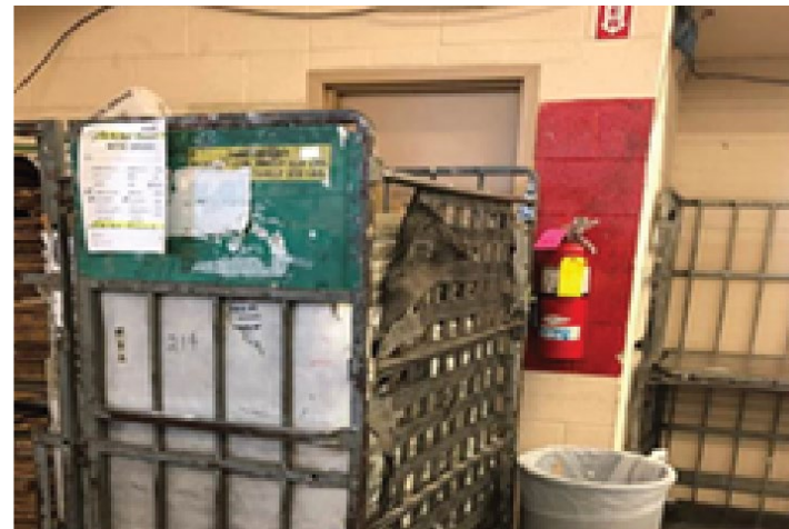
Figure 11. Blocked Inspection Service Door
