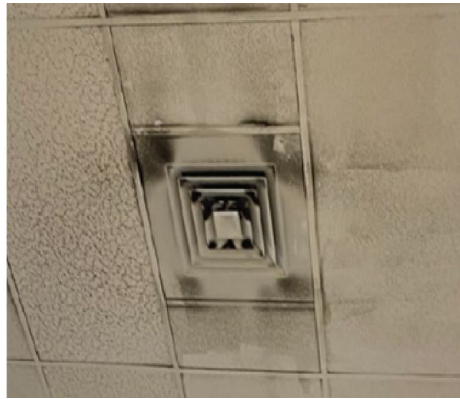
Dirty diffuser at Concord Main Post Office, Concord, MA. Photograph taken on September 22, 2021.
